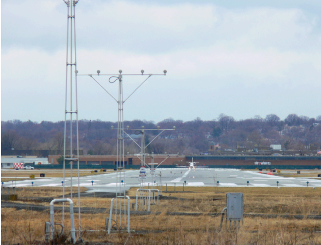
Figure 1. MALSF Runway Approach Light System (A.A. Trani).
