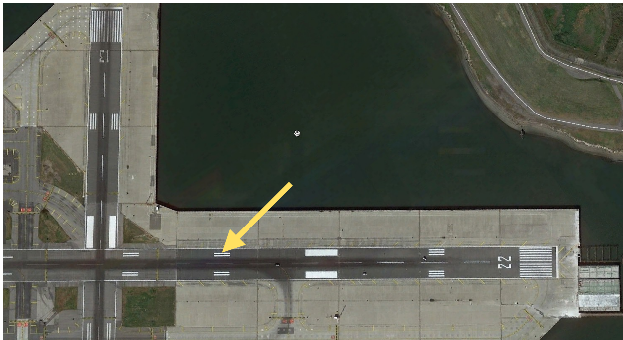
Figure 1. Configuration of LGA Airport Runways for the Problem. Arrow Points to the Area Where Landing Aircraft Main Landing Gear Touches Down.
